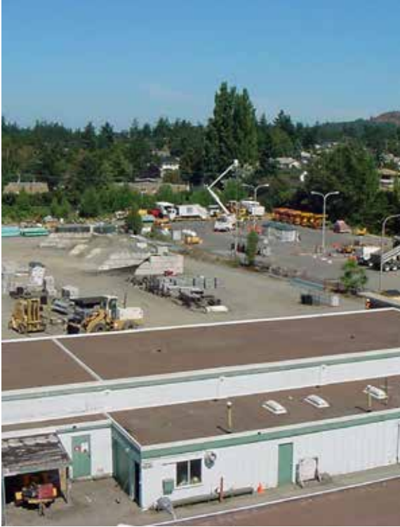
Saanich Public Works yard
