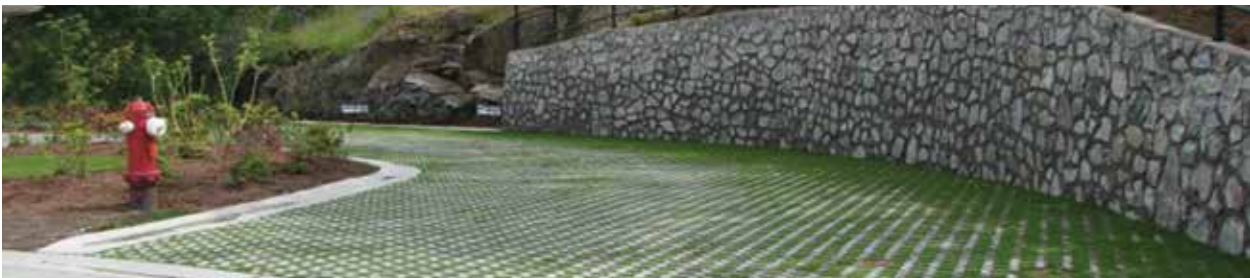
Stormwater Management ~ South Wilkinson Valley
